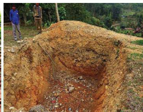
Earth excavation for WHS construction, Sanglu
