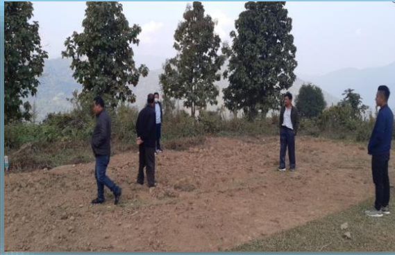
DMU Dimapur, Piphema Old Village: Nursery site Inspection, Levelling and distribution of building material for the nursery.
