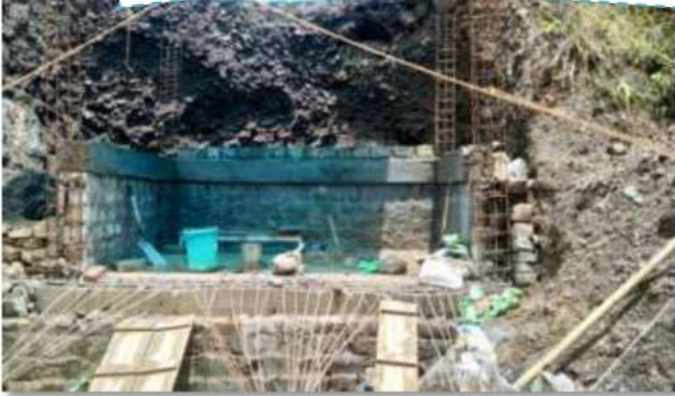
WHS at Kami Village, Phek (under construction)
