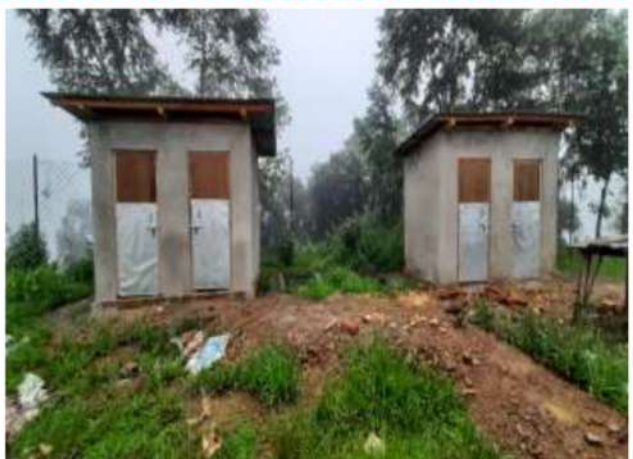
Construction of Community Toilet at Zhadima, Kohima
