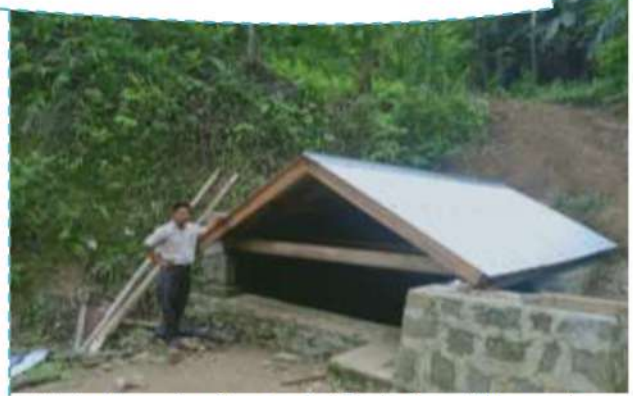
Water Harvesting Structure) at Thekrejuma Village under Piphema Beat
