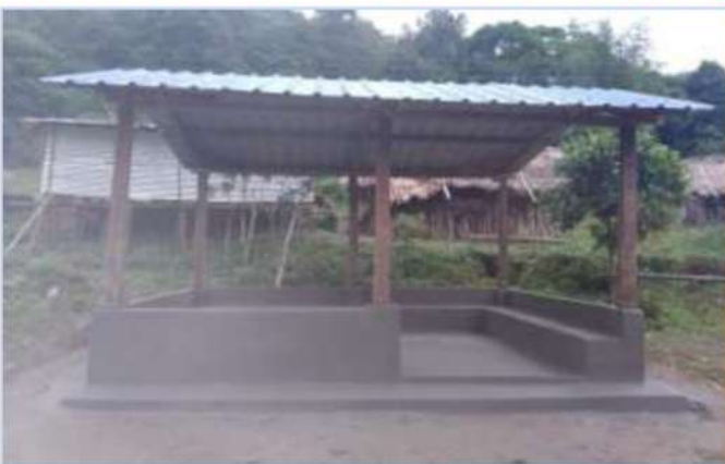
Waiting Shed (EPA) at Wanching Village, Mon
