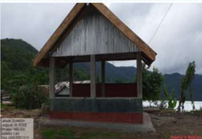
Construction of marketing shed at Tuophema village, Kohima
