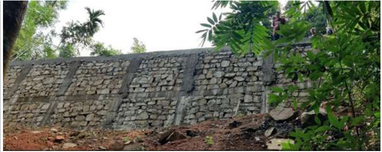
Retaining Wall renovation works at Medziphema Village (Completed)
