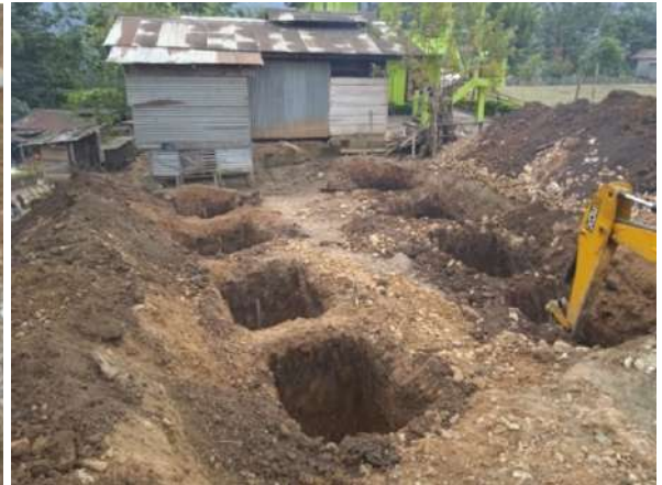
Sukomi village EPA : Community Kitchen Under Construction
