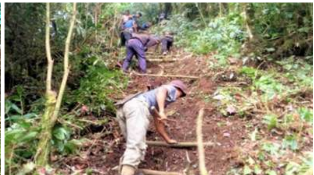
Hukphang villagers constructing Trekking Path at PEC Site.
