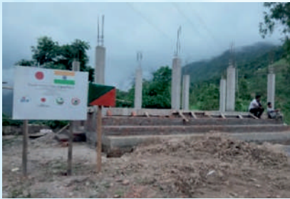
Construction of Water Harvesting Structure (WHS) at Piphema Old Village (Batch-II)
