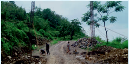
Construction of Welcome Gate (EPA) at Piphema Old Village (Batch-II)
