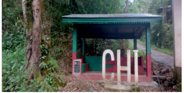
Waiting Shed (EPA) at Chi Village
