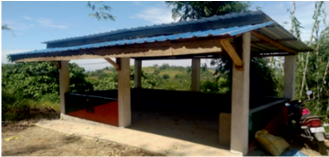
Waiting Shed (EPA) at Lampong Sheanghah
