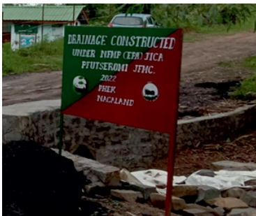
Drainage Construction (EPA) at Pfutseromi Village under EPA
