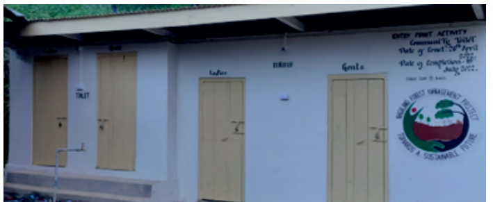
Community Toilet (EPA) at Meluri Village
