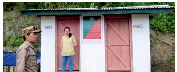
Community Bathroom (EPA) at Phenwhenyu Village
