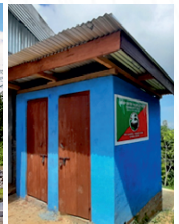
Community Toilet (EPA) at Kandinu village
