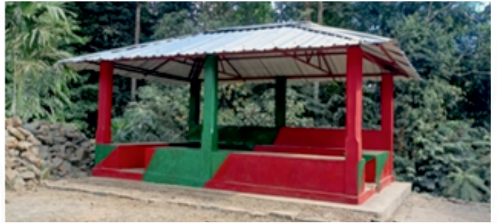
Waiting Shed (EPA) at Tanhai Village
