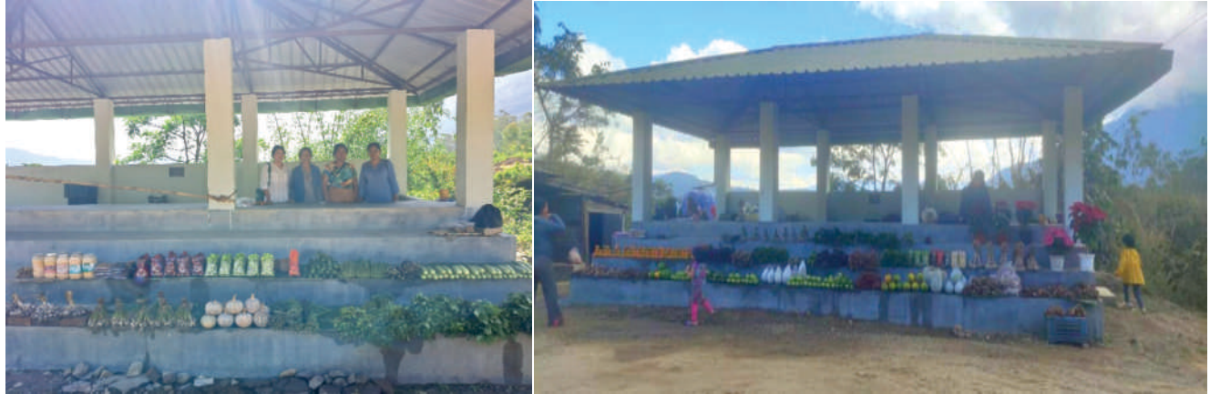
FNGO Team with Women Vendors at Piphema Old Marketing Shed cum Water Harvesting Structure constructed under NFMP JICA.
