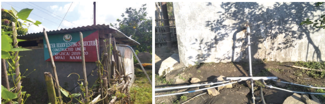
Water Harvesting Structure at Mpai Namci village.
