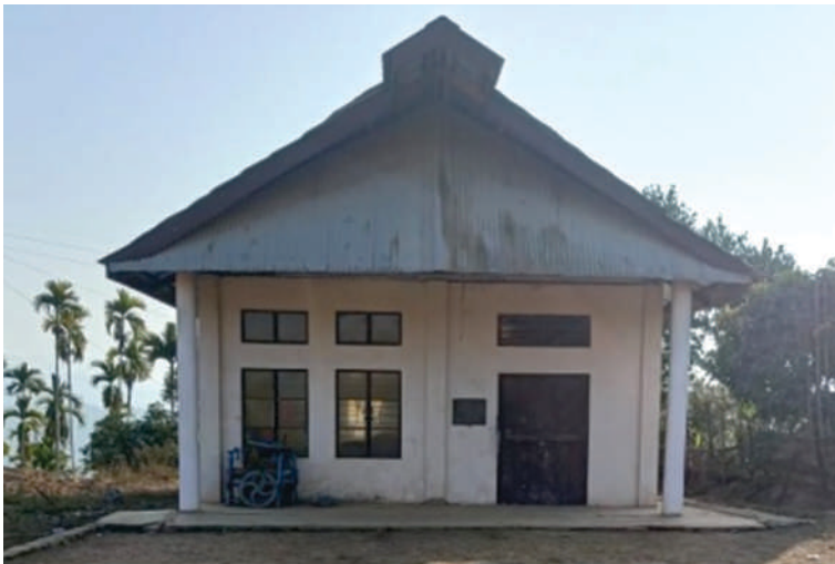
Before Construction, Kelingmen
