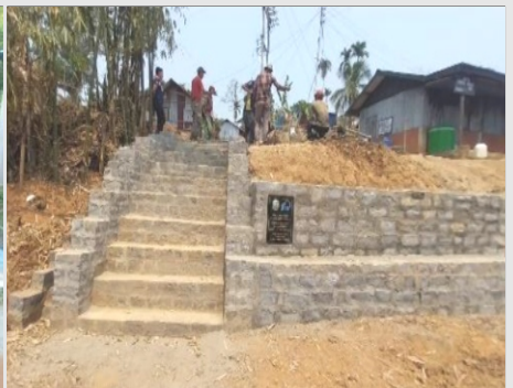
Footsteps constructed under EPA in New Changsu Village (Batch-III)
