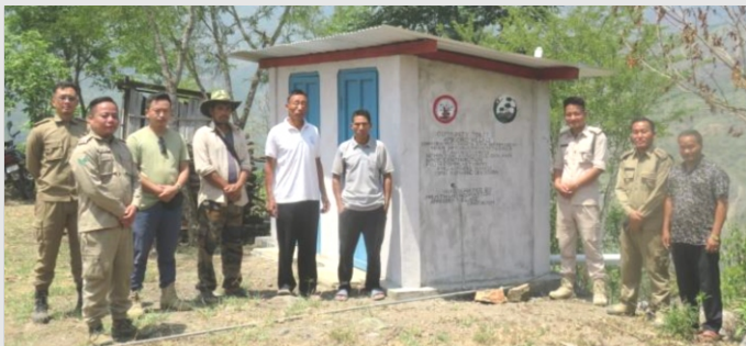
Community Toilet (EPA) of Amikiroo village (Batch-III)
