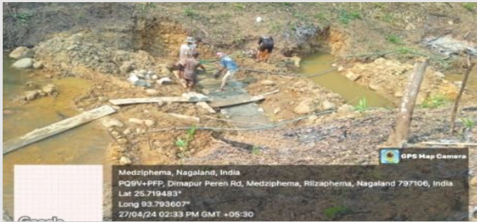
Construction of Check dam (EPA) at Ruzaphema Village (Batch-III) was completed on 25 th May 2024. The check dam measures 30ftx3ftx7ft (lwxhx)
