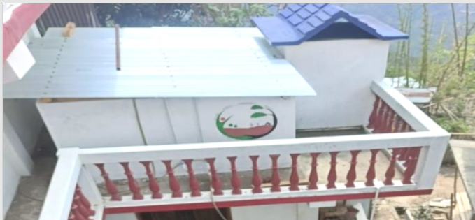
WHS at Phusachodu Village
