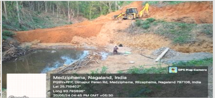
Construction of Check dam (EPA) at Ruzaphema Village (Batch-III) was completed on 25 th May 2024. The check dam measures 30ftx3ftx7ft (lwxhx)
