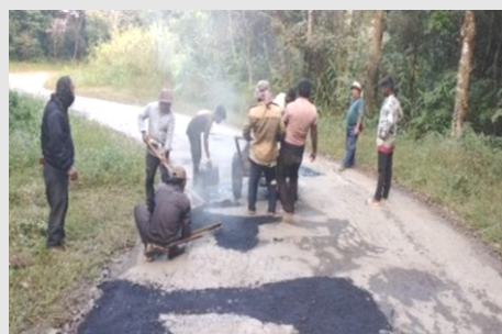
Black topping of road at Longkhum village
