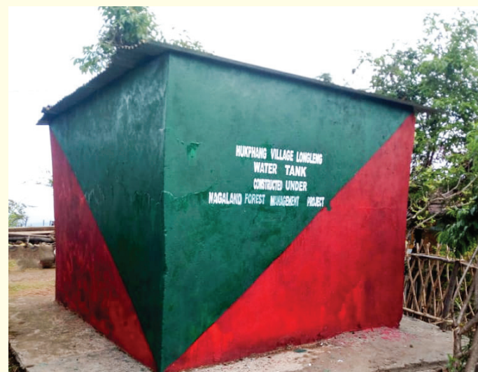
WHS constructed in the village
