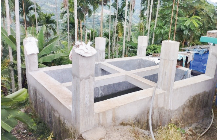
Water storage tank under construction
