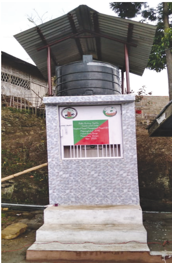
Public drinking water facility at Mopungchuket village
