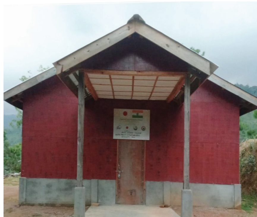
Community Hall constructed under EPA at Akhen village
