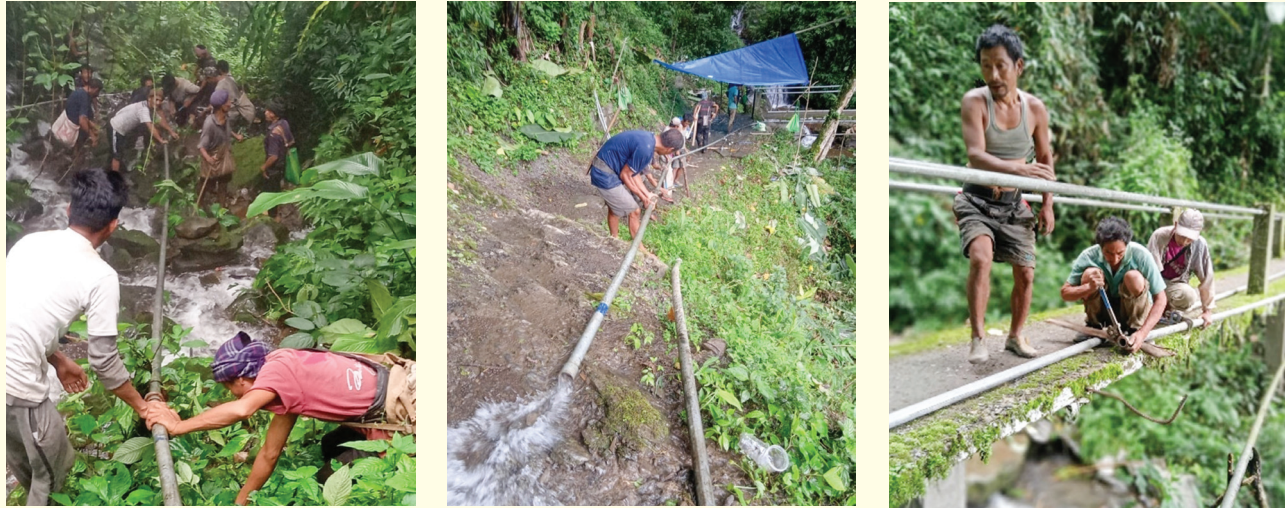
Community members of Hukphang village installing pipelines from the water source
