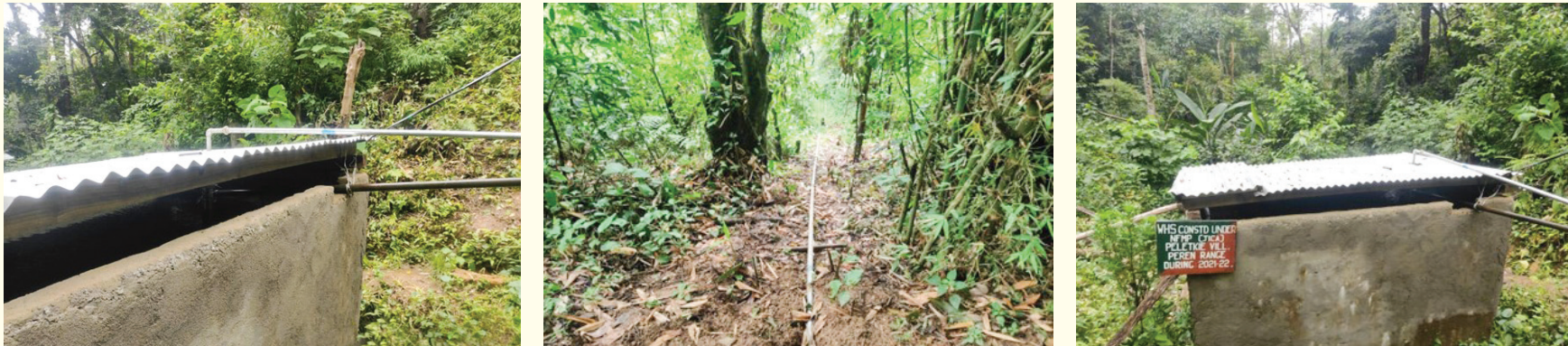
Completed Water Harvesting Structure (WHS) and pipelines at Peletkie village
