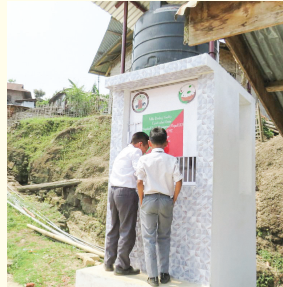
School students utilizing the drinking water facility
