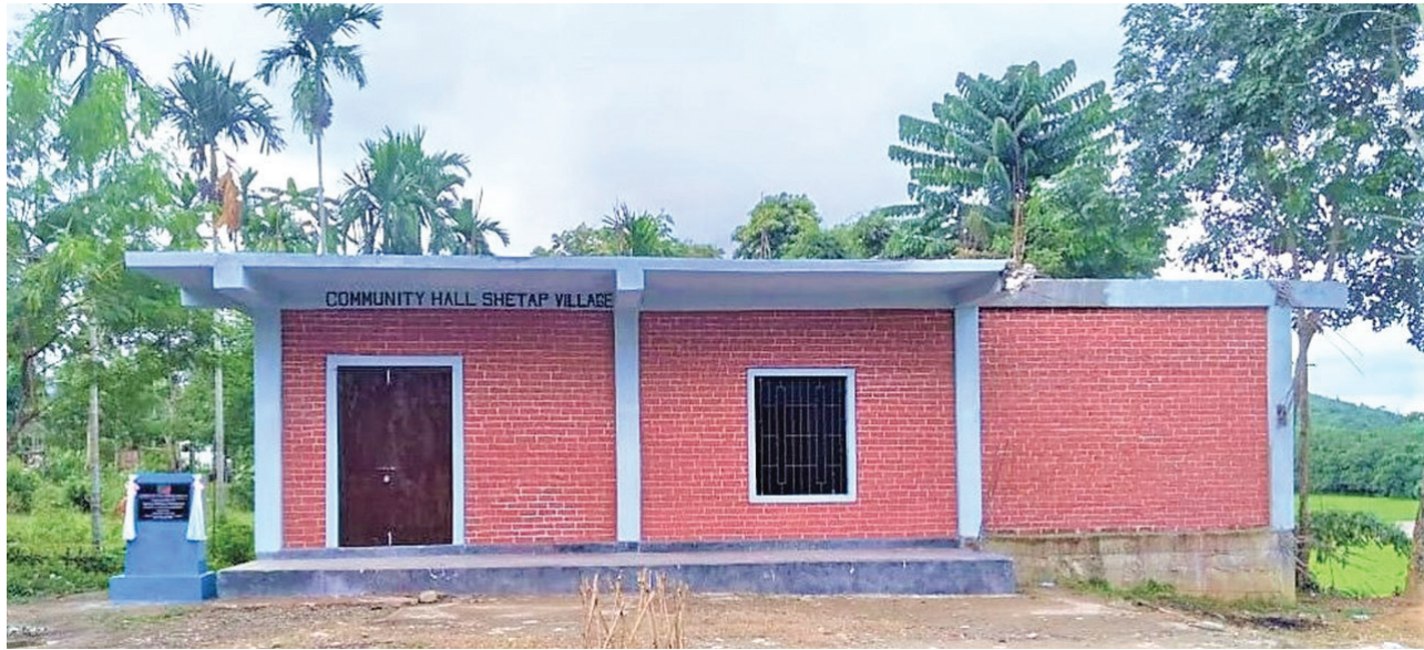
Community Hall constructed as an EPA at Sitap village
