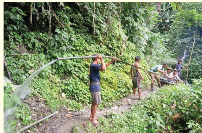
Community members of Hukphang village installing pipelines from the water source
