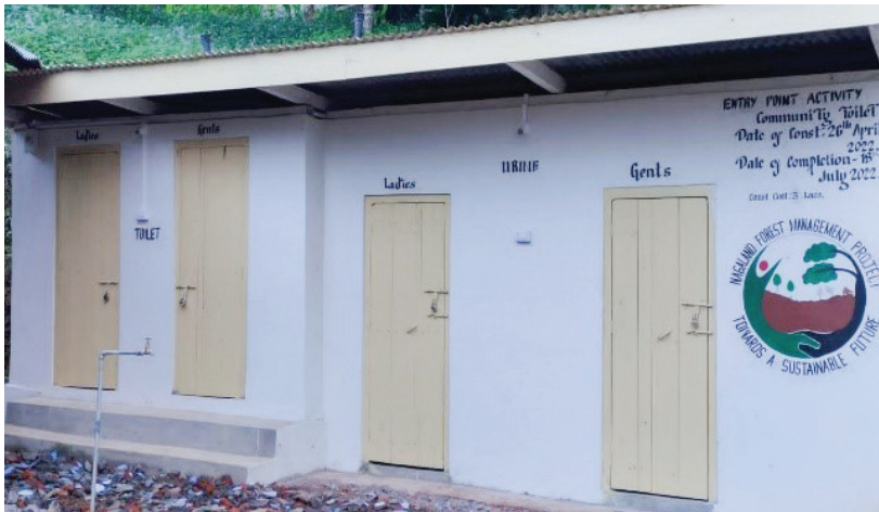
Toilet constructed under EPA at Meluri
